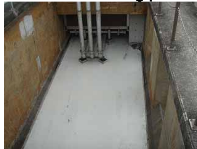
After flushing process
