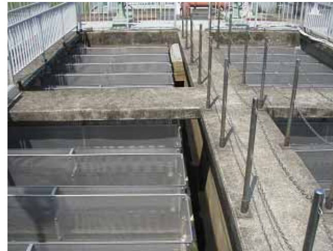
Filtration sect. (upside)
